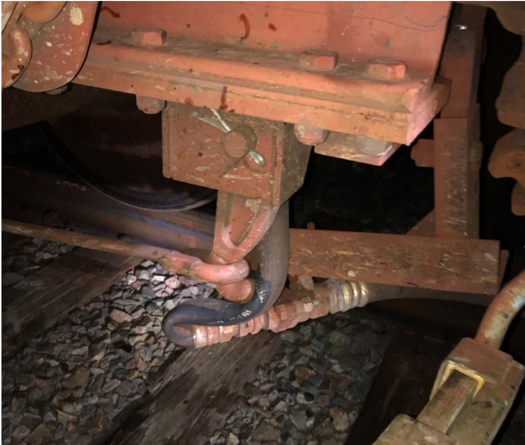
Figure 1. Kinked end-of-railcar air hose on railcar brake rigging of train involved in the November 23, 2018, incident west of Cheyenne, Wyoming. (Photograph provided by UP.)
