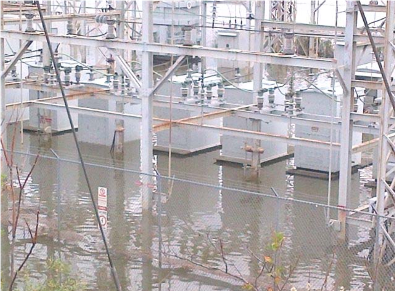
Limited traffic between Newark and NYC due to constrained power availability
