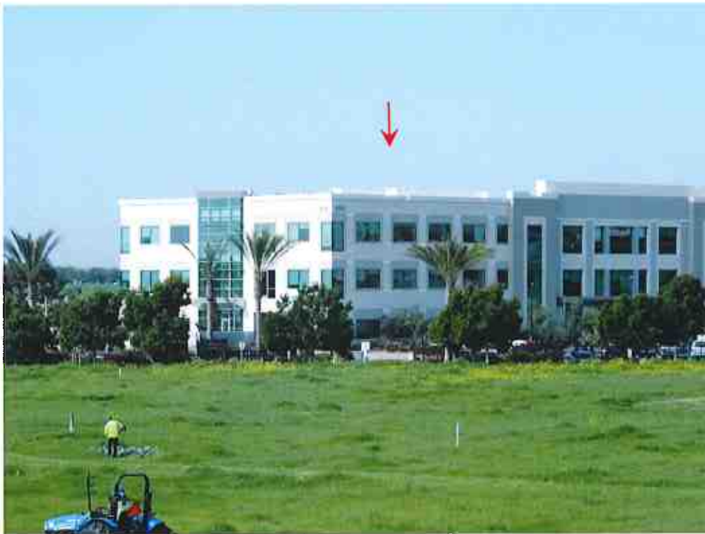
View toward TX antenna on rooftop from Site 7 at 10m AGL (zoom)
