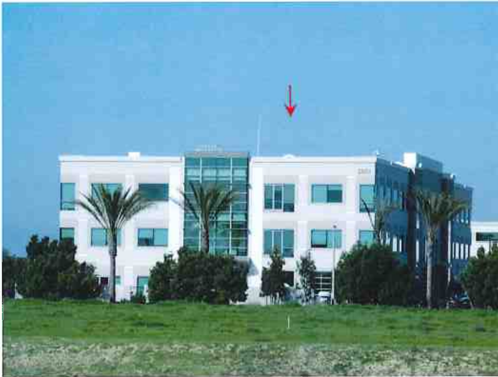
View toward TX antenna on rooftop from Site 9 at 10m AGL (zoom)
