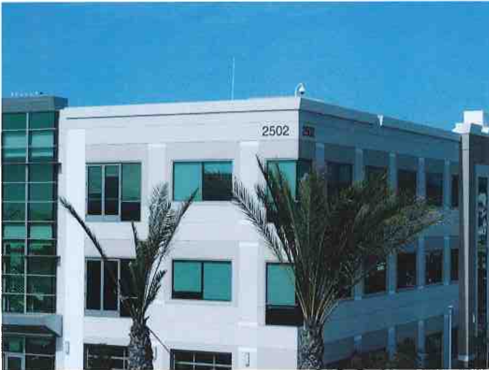
View toward TX antenna on rooftop from Site 2 at 10m AGL (zoom)
