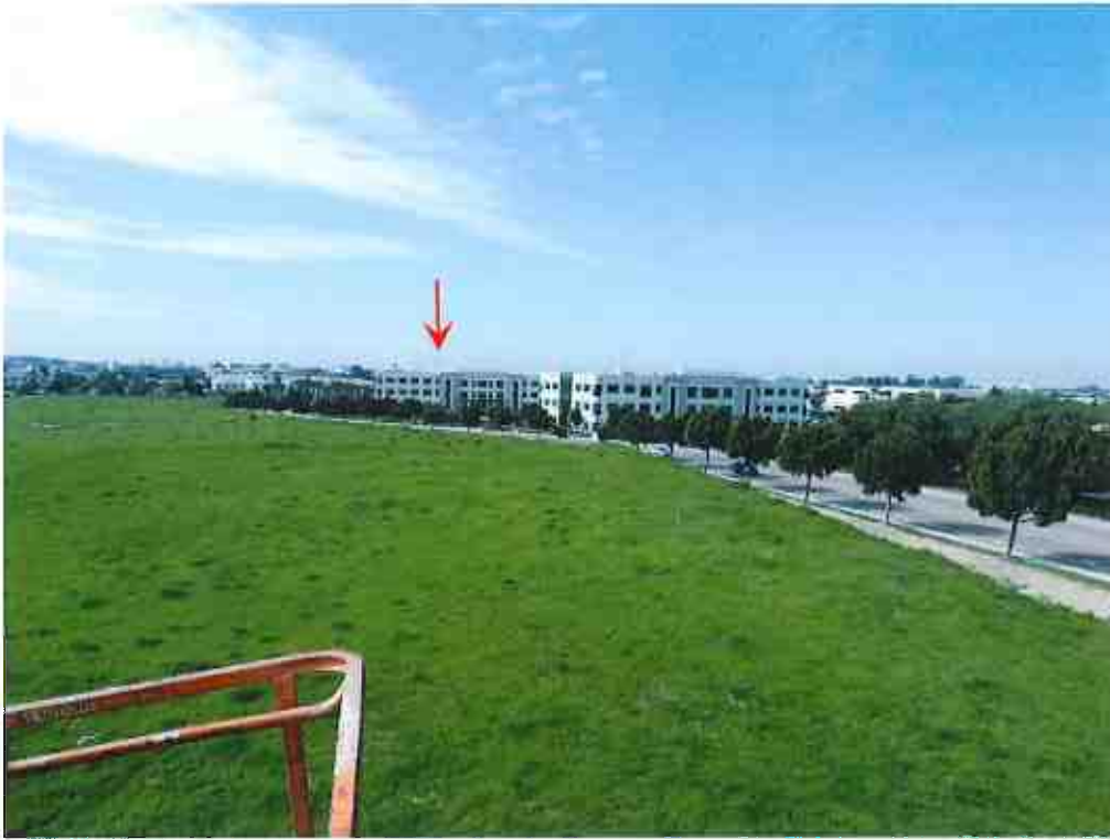
View toward TX antenna on rooftop from Site 5 at 10m AGL
