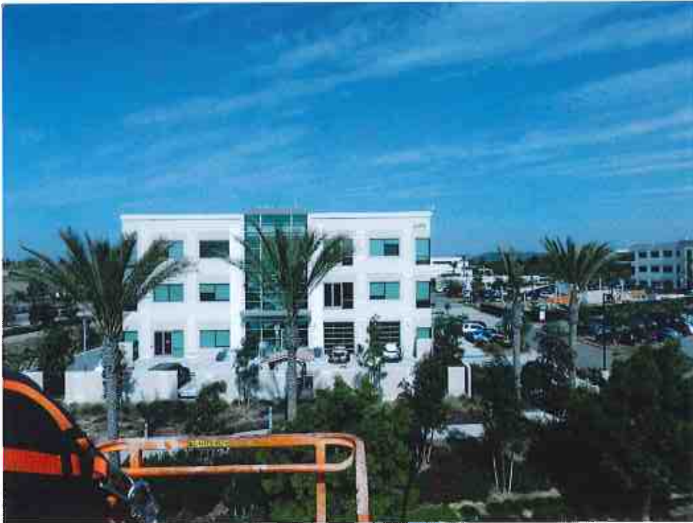
View toward TX antenna on rooftop from Site 1 at 10m AGL
