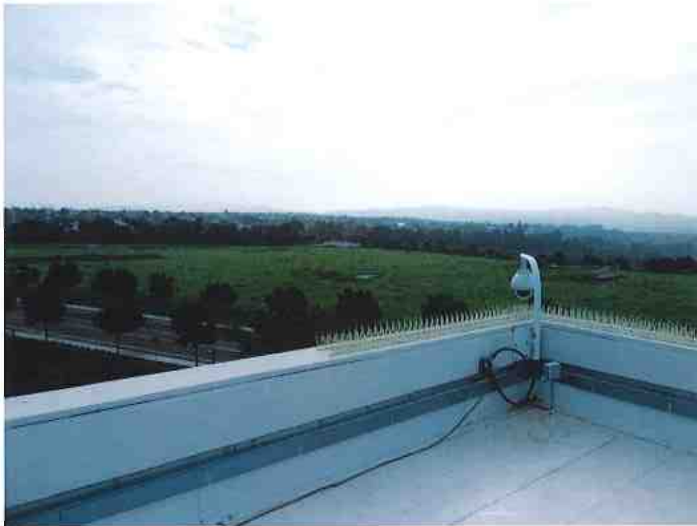
View from rooftop looking southeast
