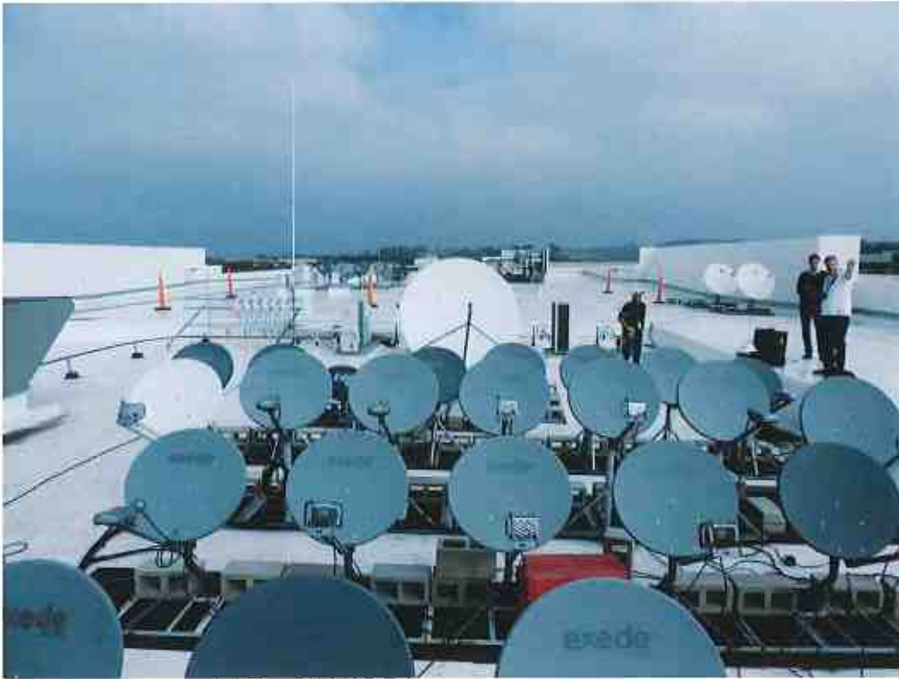
View of transmit antenna looking north
