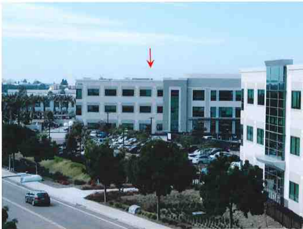
View toward TX antenna on rooftop from Site 4 at 10m AGL (zoom)
