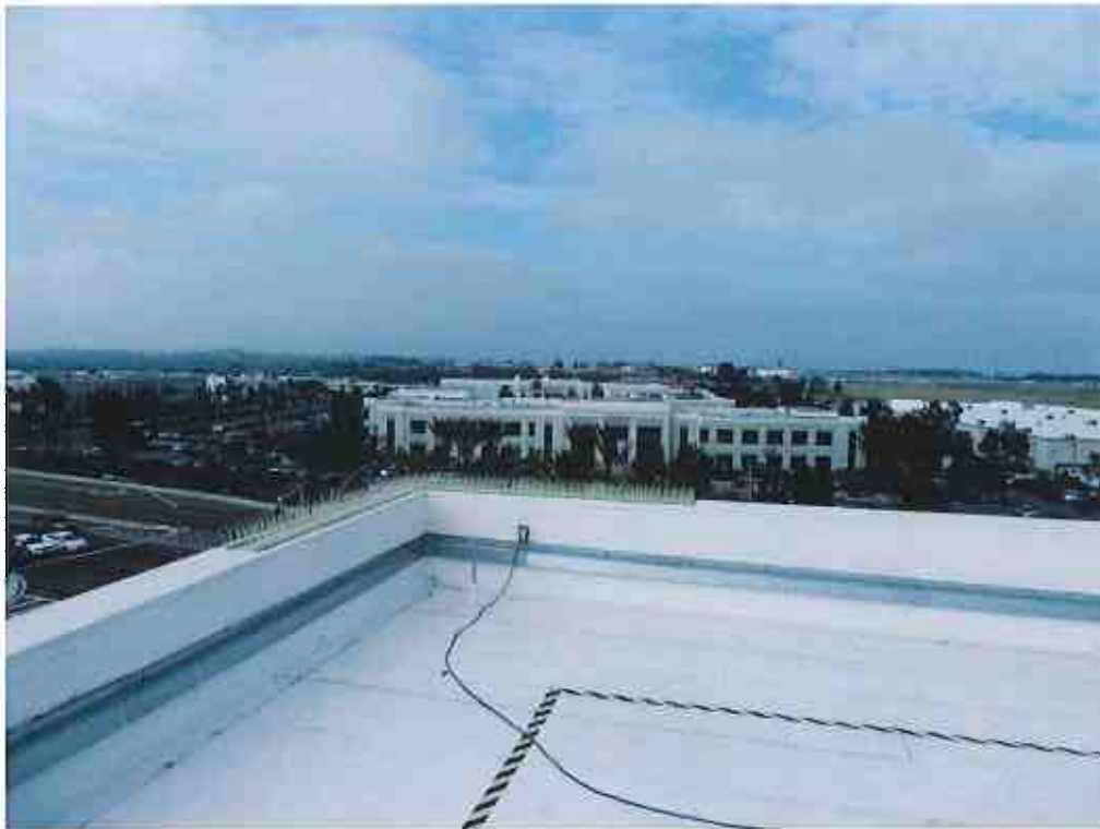
View from rooftop looking southwest
