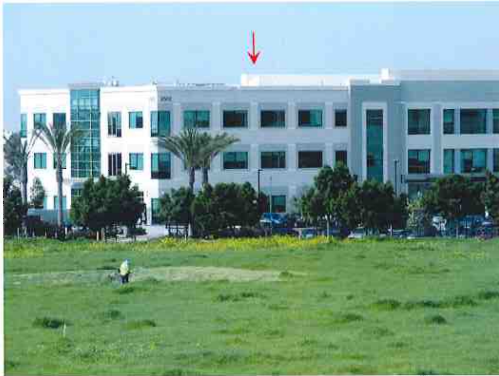
View toward TX antenna on rooftop from Site 6 at 10m AGL (zoom)
