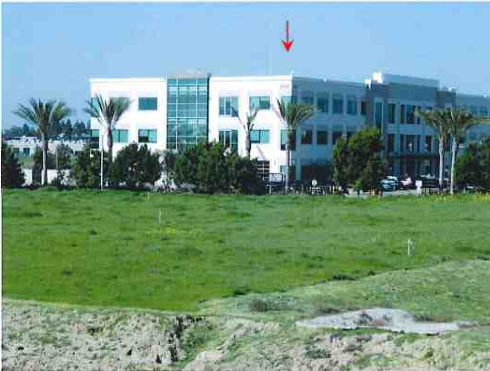
View toward TX antenna on rooftop from Site 8 at 10m AGL (zoom)
