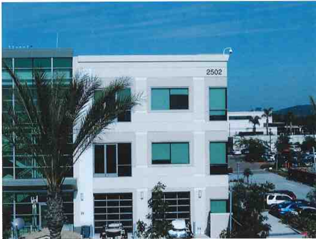
View toward TX antenna on rooftop from Site 1 at 10m AGL (zoom)
