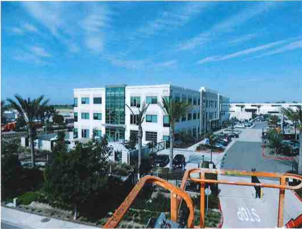
View toward TX antenna on rooftop from Site 2 at 10m AGL
