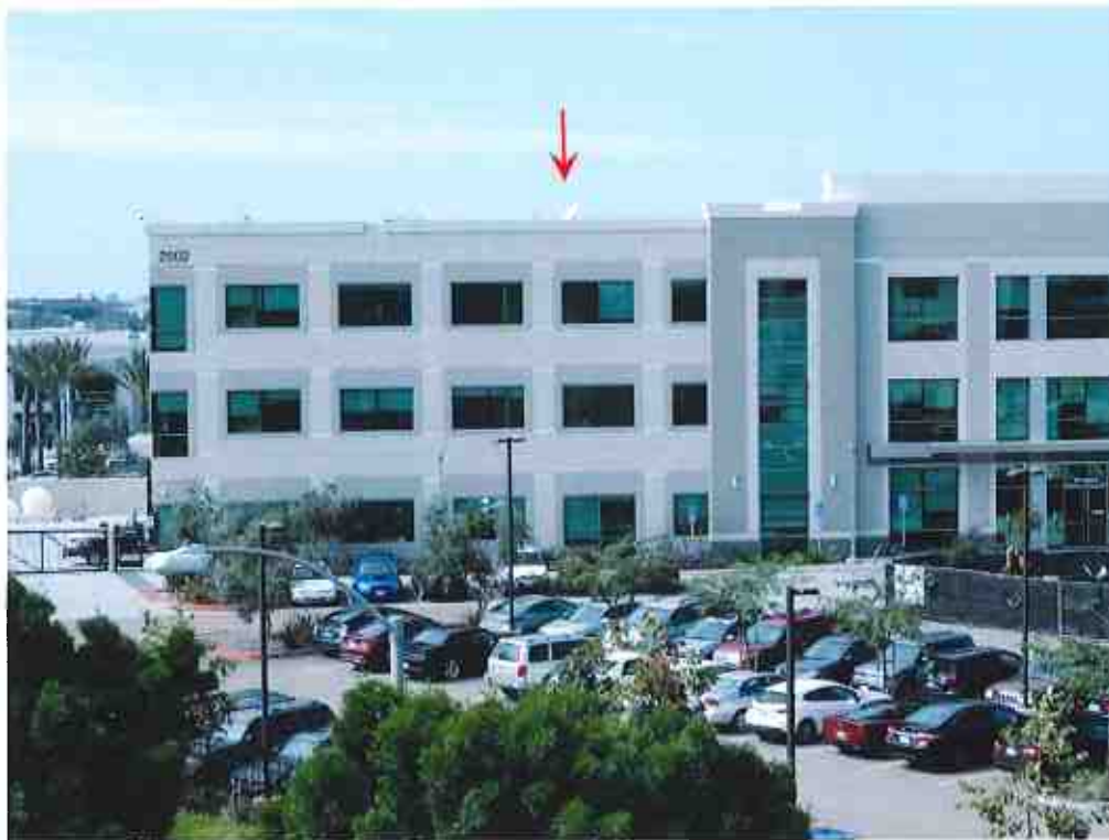
View toward TX antenna on rooftop from Site 3 at 10m AGL (zoom)
