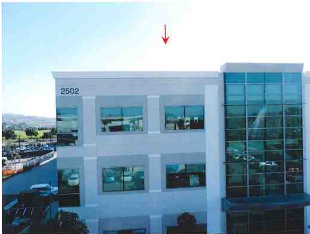
View toward TX antenna on rooftop from Site 11 at 10m AGL (zoom)
