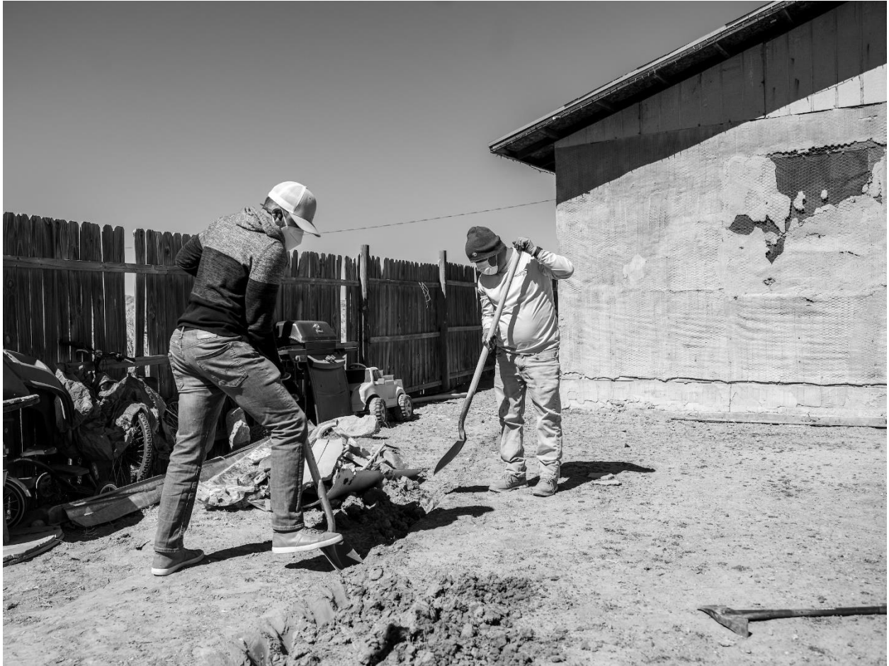
Starlink setup, digging trench
