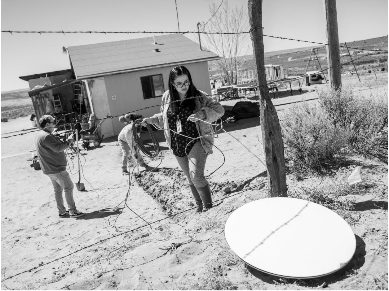
Starlink setup, running cables
