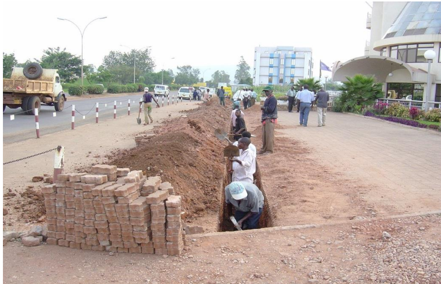
Figure 2: Fiber installation in 2003 in Kigali, Rwanda
