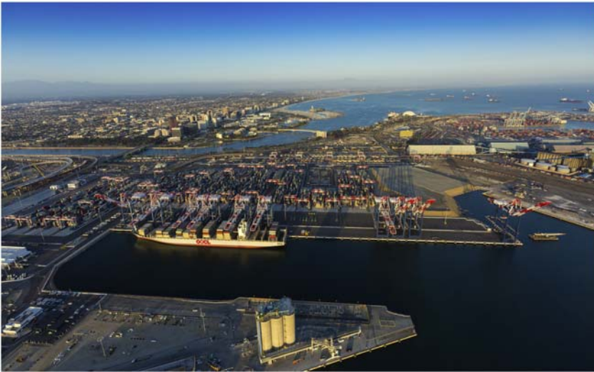
Figure 4.1 Equipped with nearly all electric- and zero-emissions technologies, the Port of Long Beach’s Middle Harbor Terminal is one of the most environmentally sustainable container terminals in the world.
